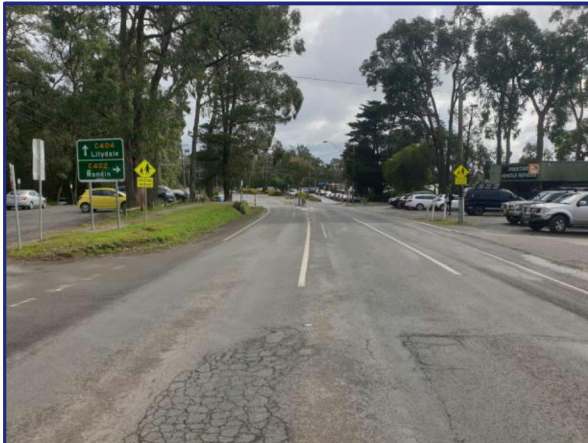
Figure 5: Monbulk Road view North
